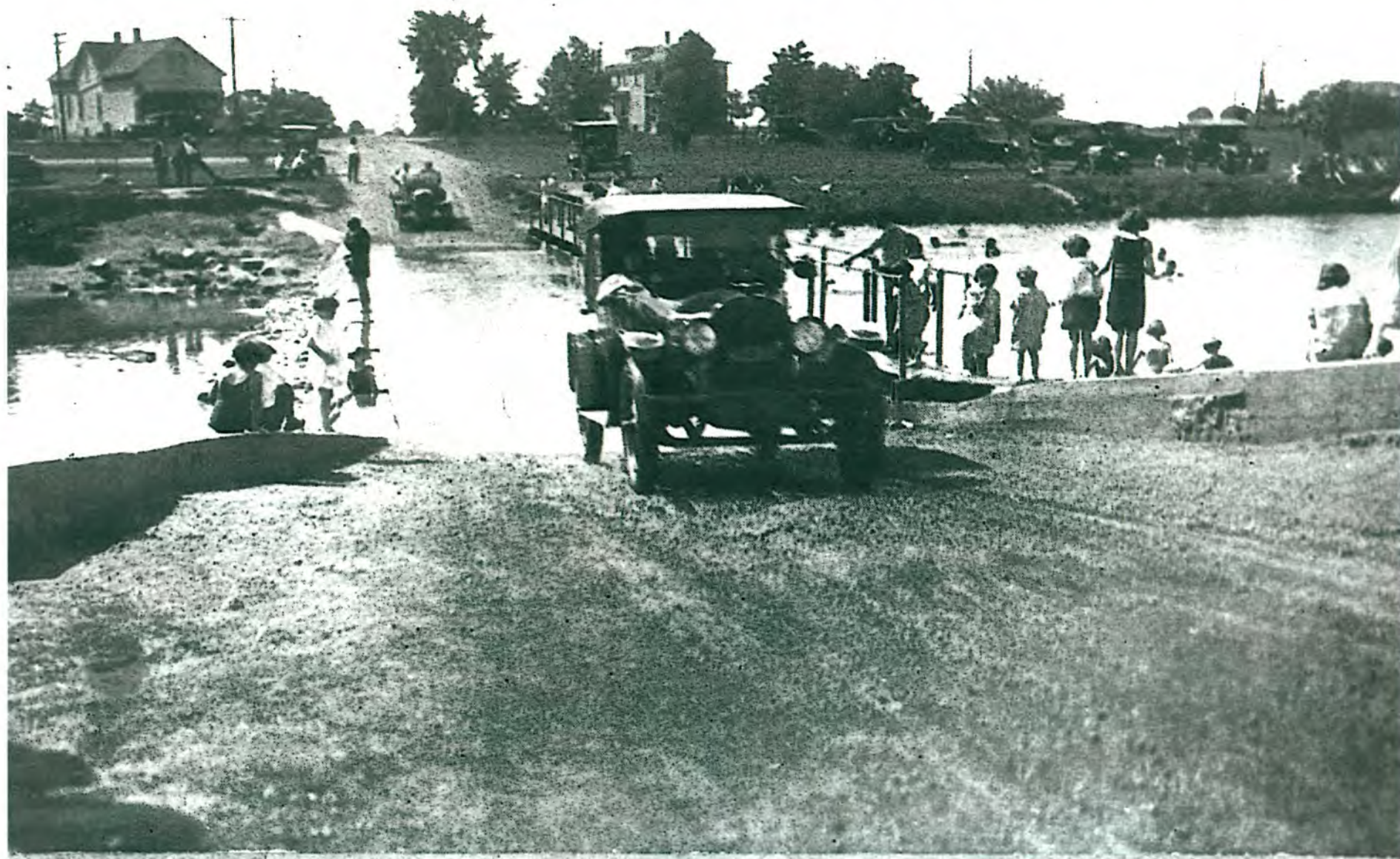
Looking West across Desplaines River, Dam No. 1, Cook County Forest Preserve Wheeling, Ill. 49706-nr
