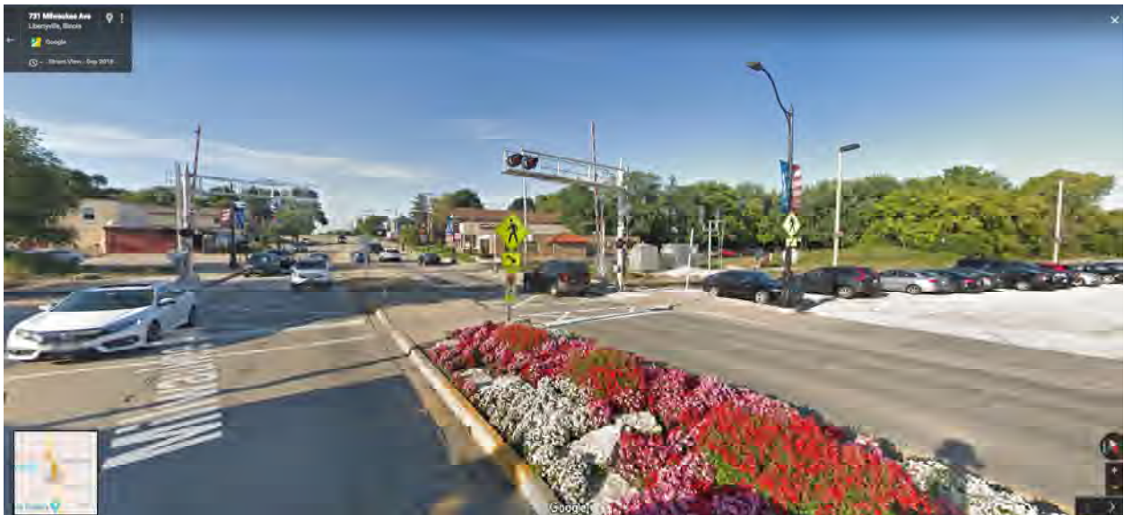
NCS rail crossing with pedestrian island at Milwaukee Ave. Libertyville,
