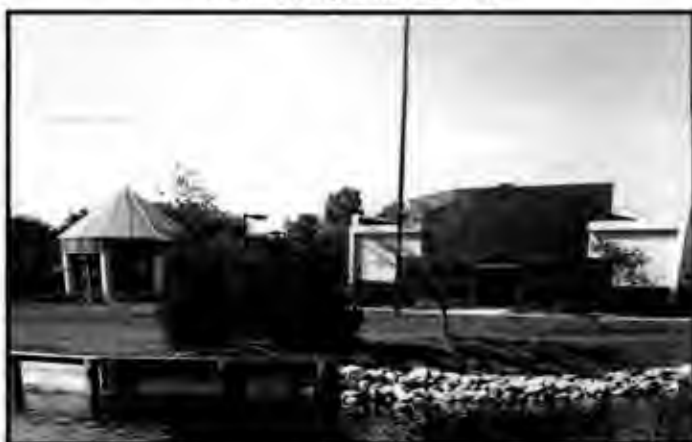
New Construction of the Pavilion and Gazebo
